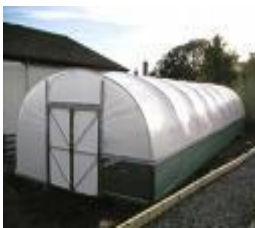
A hoop formed polytunnel
